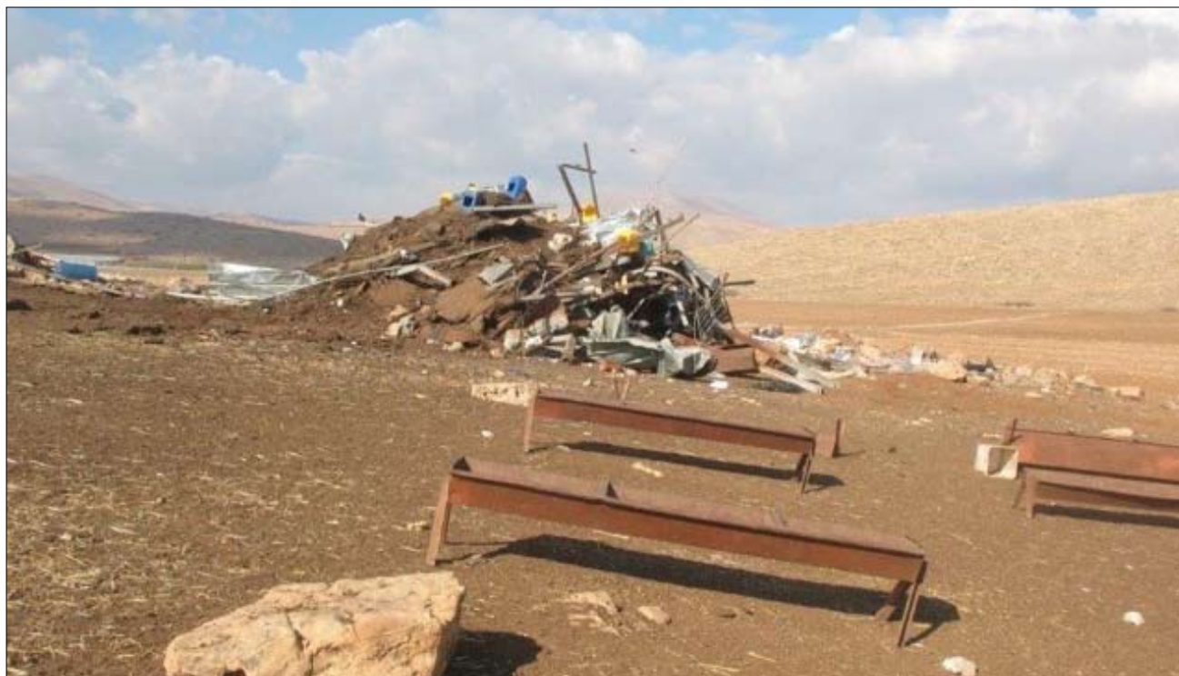
El Hadidya Demolitions, November 2015
